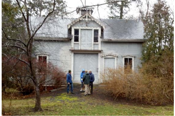
Carriage House, 21 Academy Lane, west facade
