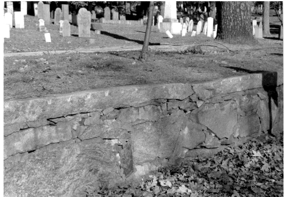
11. New Burying Ground: retaining wall, with notches for jail bars
