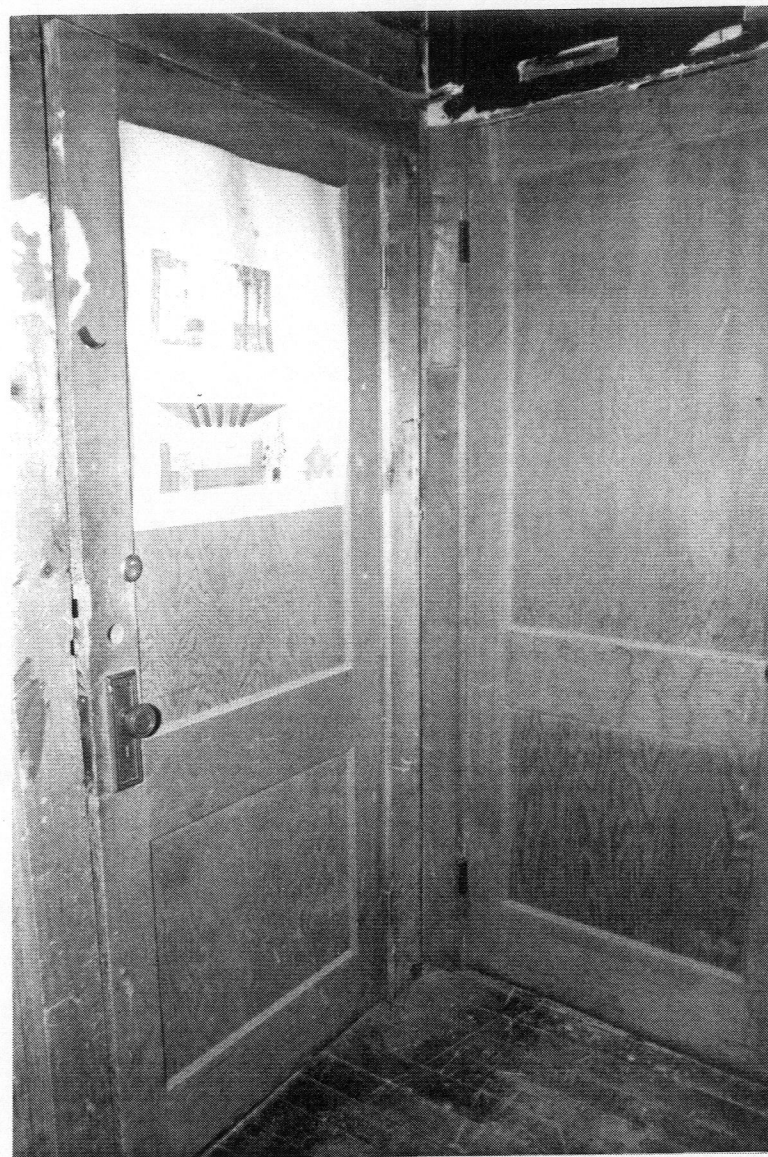
STAGES: ca. 1922 2-panel doors with face-veneer plywood
