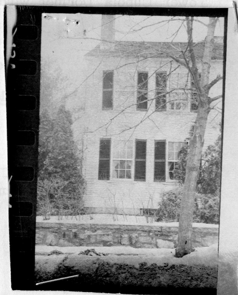
Detail to show graduated Clapboards
