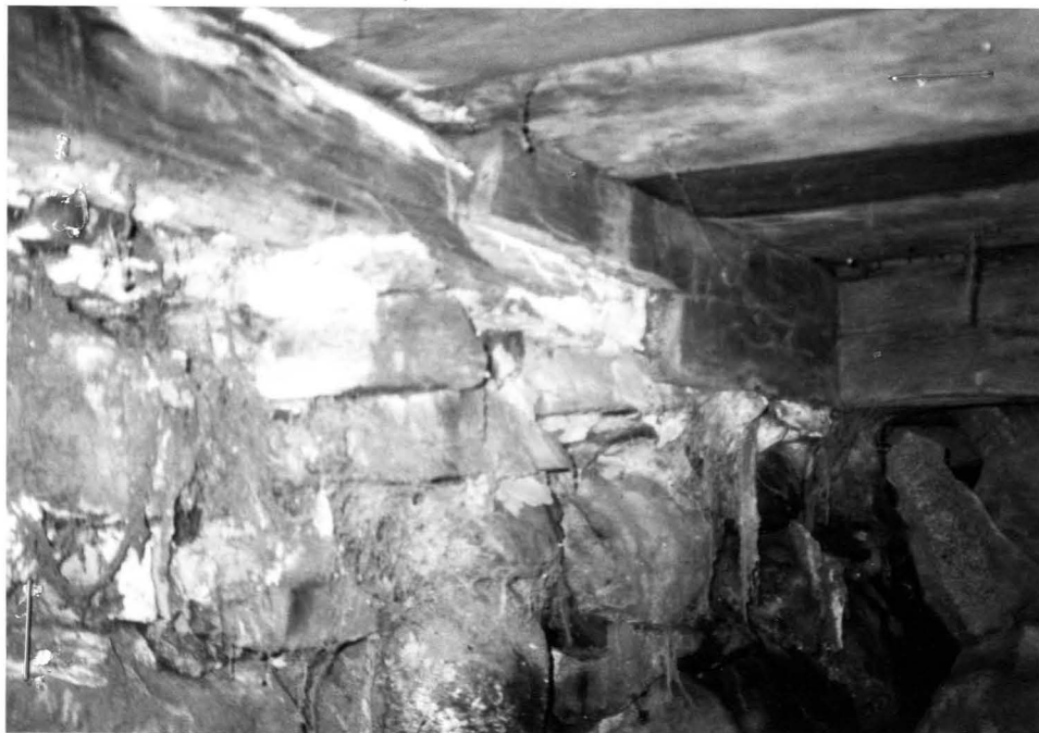
Joint in front sill
