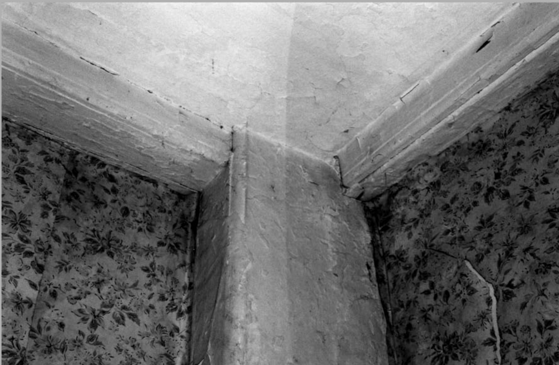
13. Second story: connection of northwest corner post, rear plate, and end girt (Photographer: Anne Forbes, August 2000)
