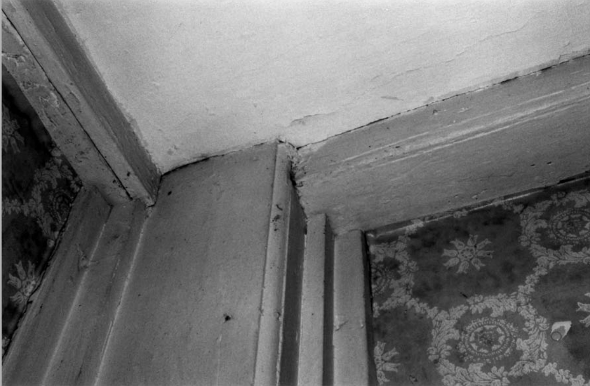
12. Second story: connection of southwest corner post, front plate, and end girt (Photographer: Anne Forbes, August 2000)
