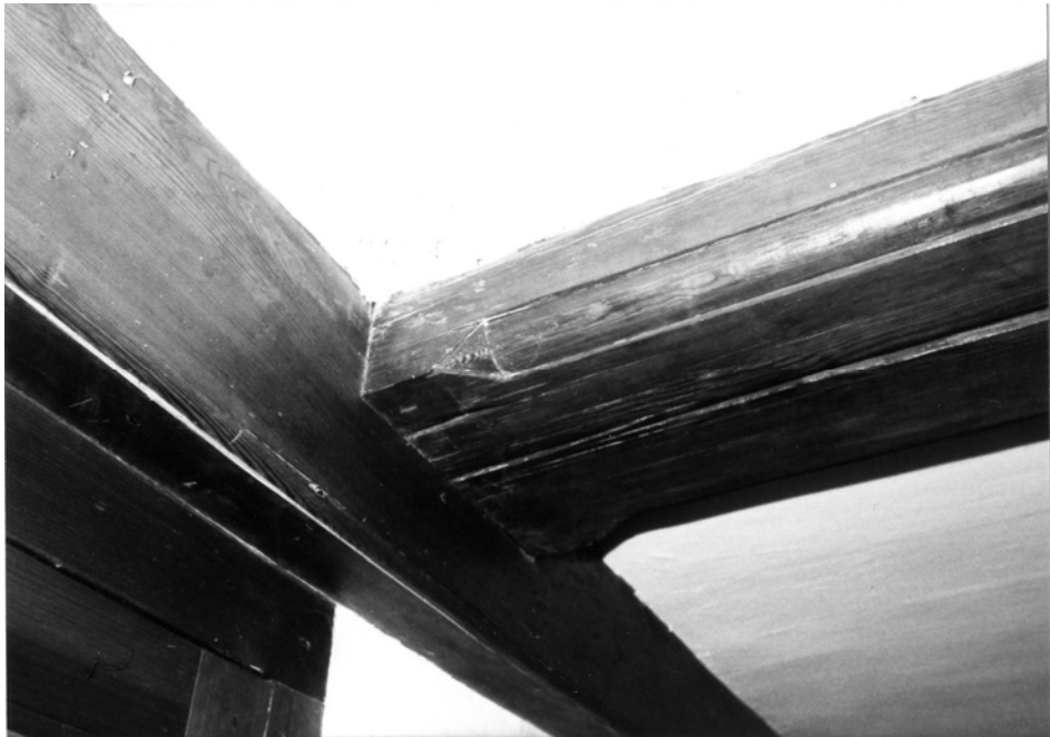
76:2A-3 Binding summer beam with quarter-round chamfer and taper stop in southeast chamber
